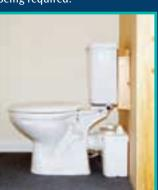
Since many close coupled WC suites do not have the space between the WC pan spigot and the wall, you may have to batten the cistern off the wall to make room for the Saniflo. However Sanislim will fit behind most closed coupled WC suites without the need for this.
